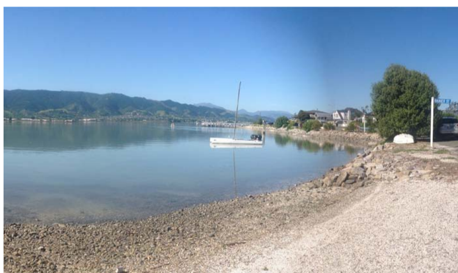
Above: Gravel and rock rip rap surrounding Monaco with coastal access extended along the edge of the urban area
