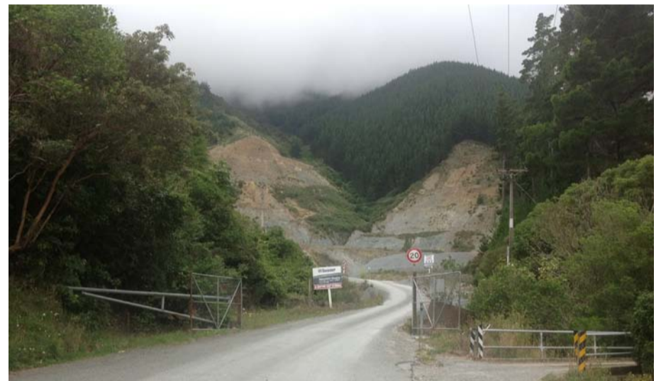
Above: Quarrying activity extended into Barnicoat Range at eastern end of Marsden Valley.
