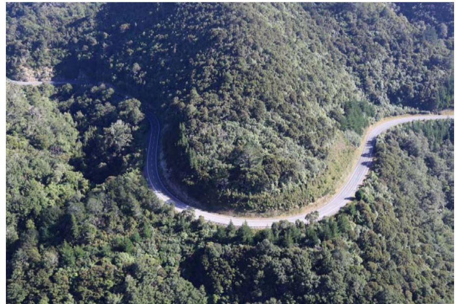
Below: State Highway 6 snakes its way through an enclosed hinterland character.
