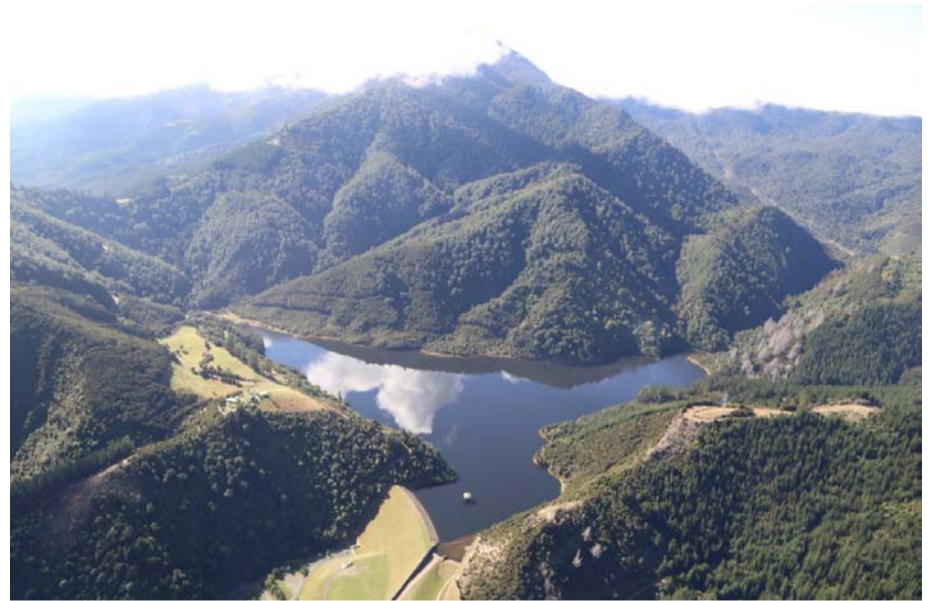
Above: Maitai Dam occupies the upper reaches of the Maitai Valley accommodating a large triangular lake accessible from the end of the Maitai Valley Road
