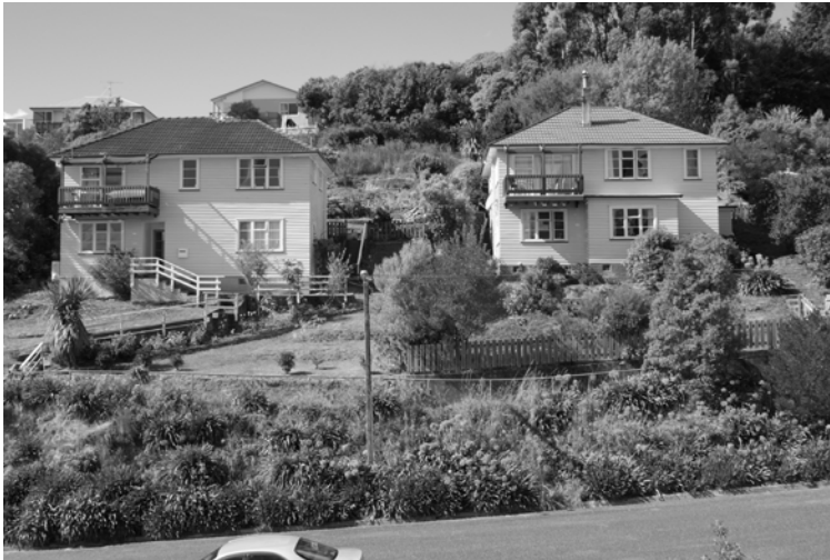
Two of the interesting group of post-war State houses on Wolfe Street.
