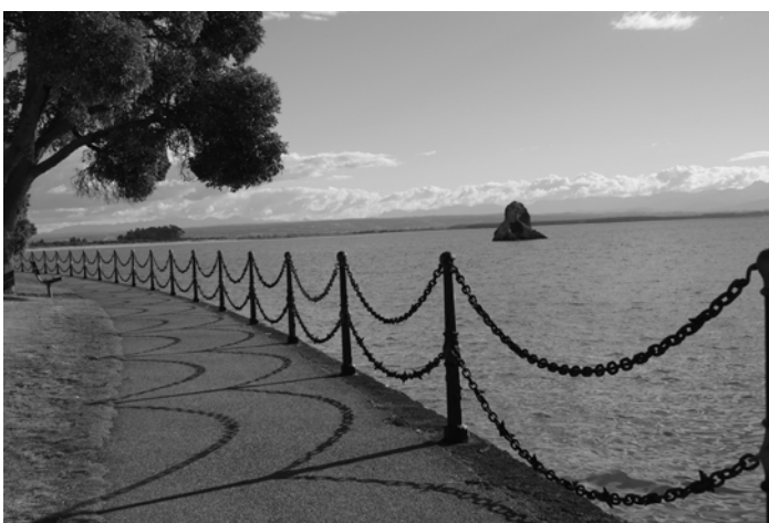
The historic chain fence along Rocks Road.
