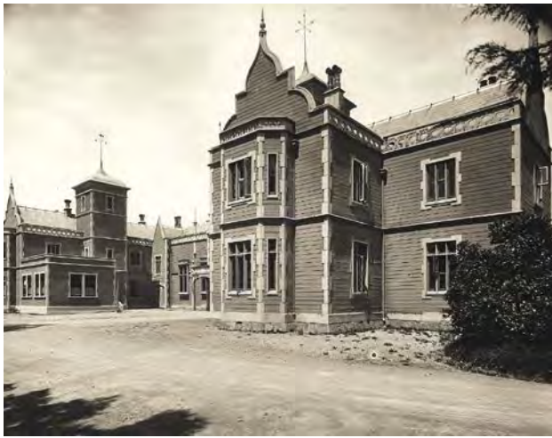
The 1969 demolition of Nelson's Provincial Government Buildings was a key incident in the development of the historic preservation movement nationwide.
