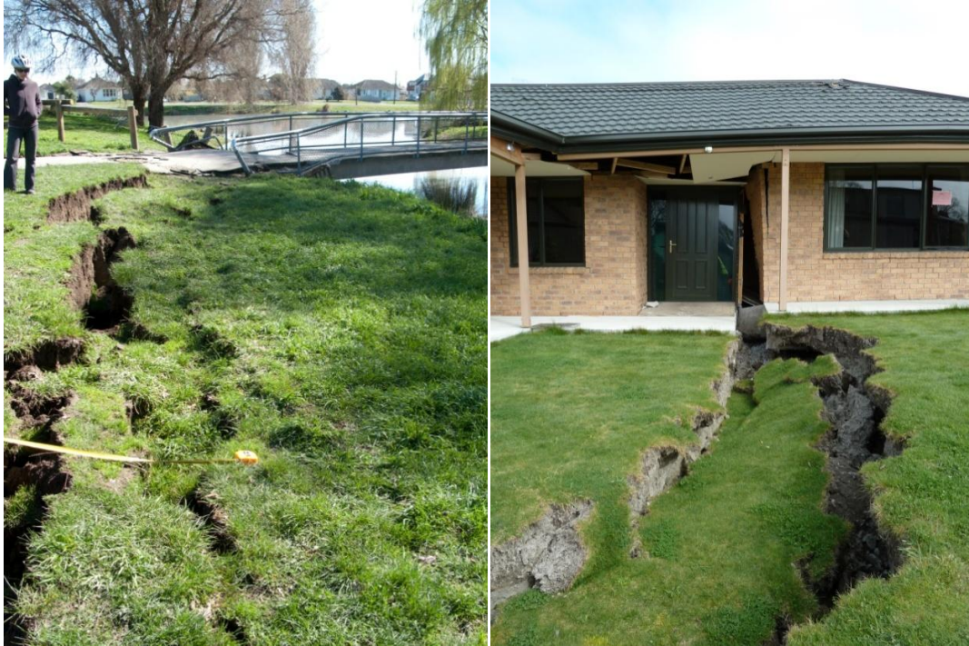
Figure B4: Lateral spreading showing horizontal and vertical displacement of land causing damage to structures
