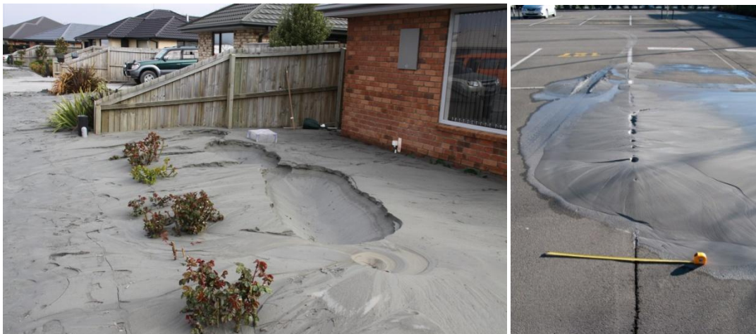
Figure B2: Surface ejection of soil and water as sand boils
