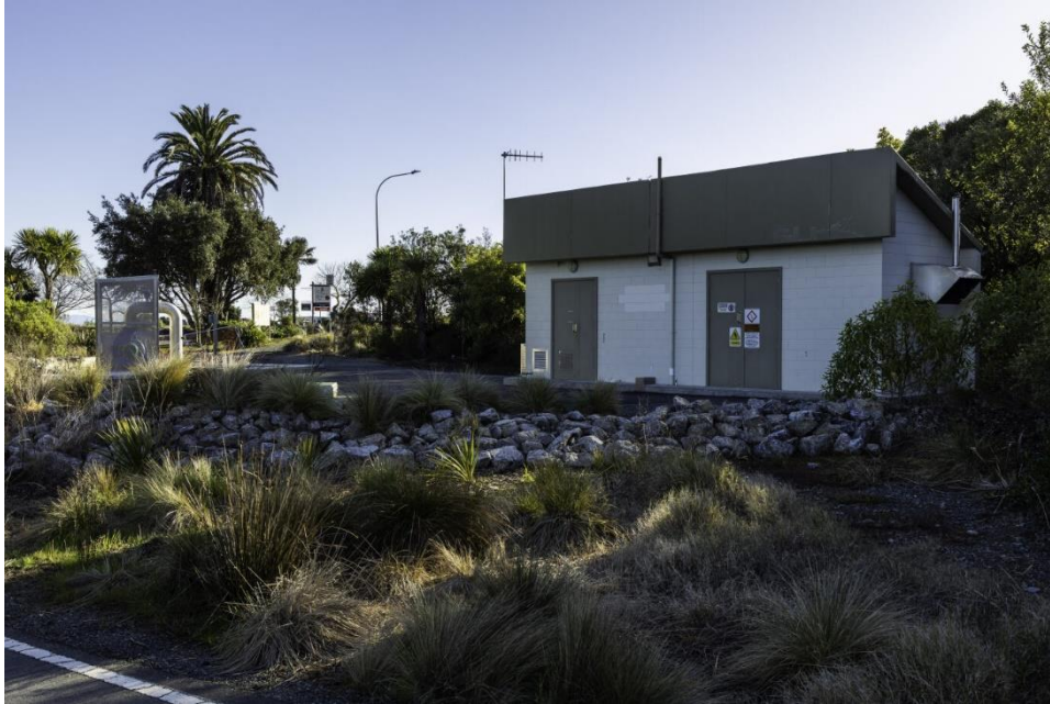
Figure 7-7: Photograph of Songer Street Pump Station site
