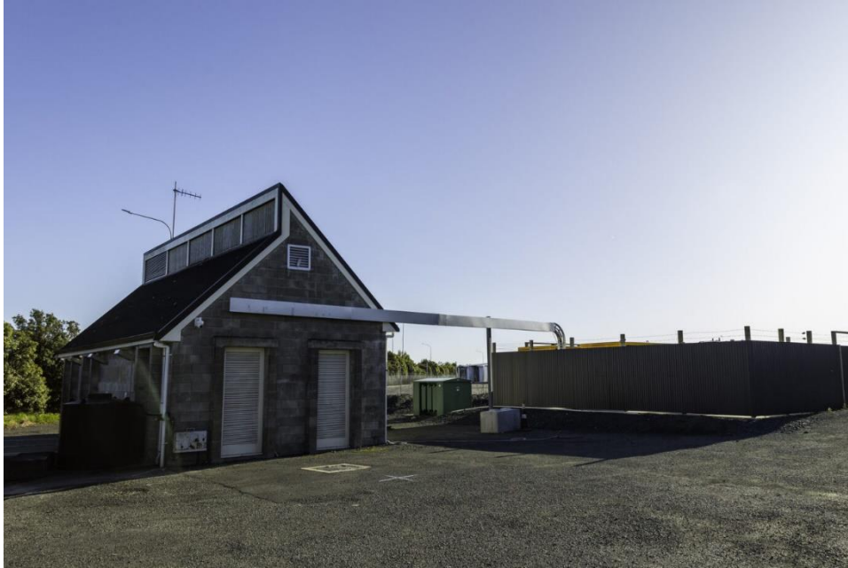
Figure 7-5: Photograph of the Saxton Road Pump Station site
