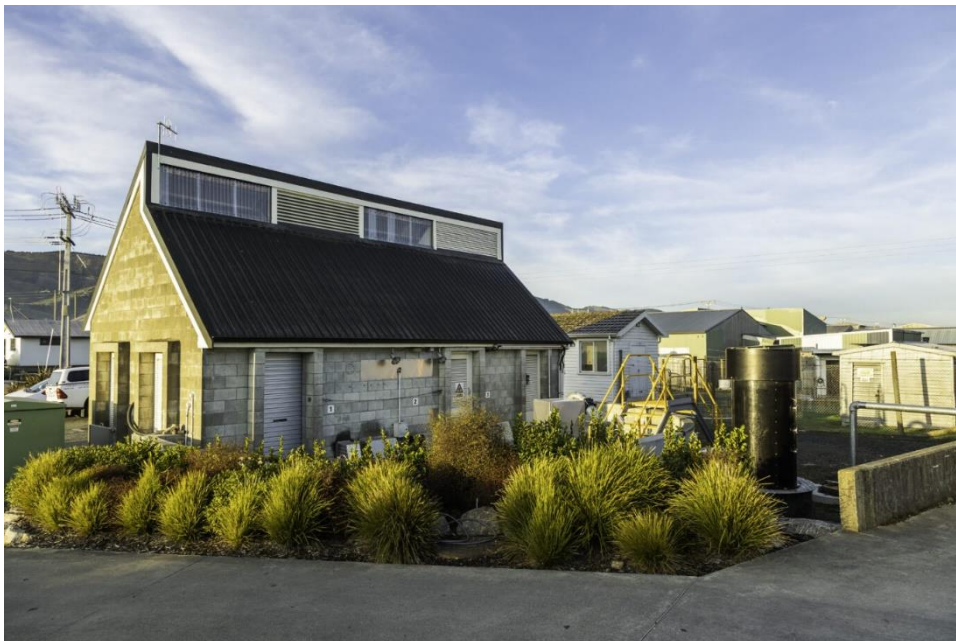
Figure 7-1: Photograph of the Beach Road Pump Station site
