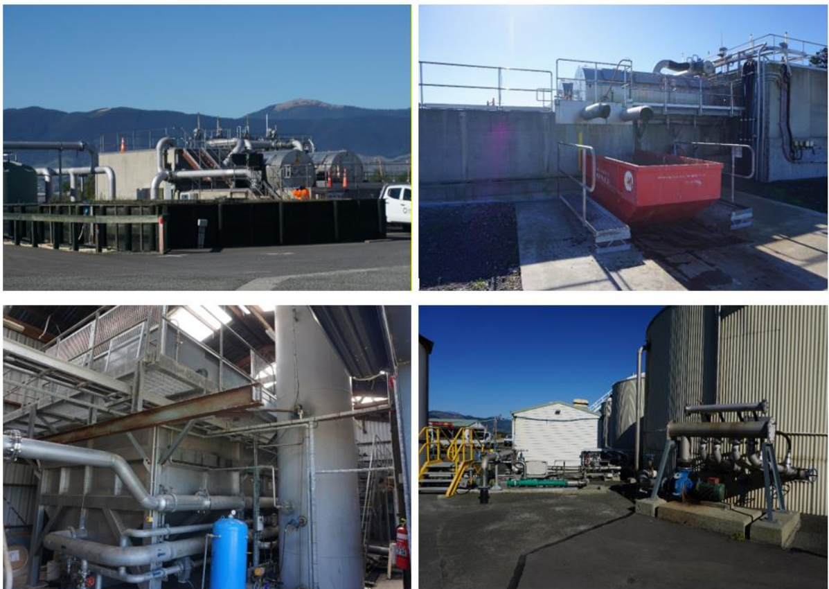
Figure 8-1: Bell Island WWTP (2022)
