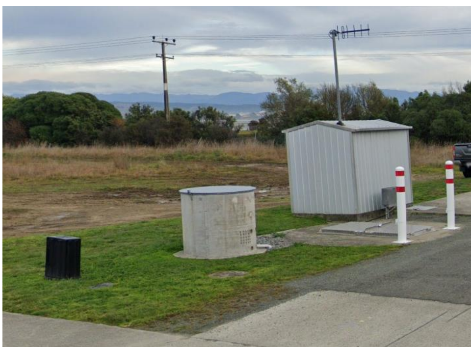
Figure 7-3: Photograph of the Wakatū Pump Station site
