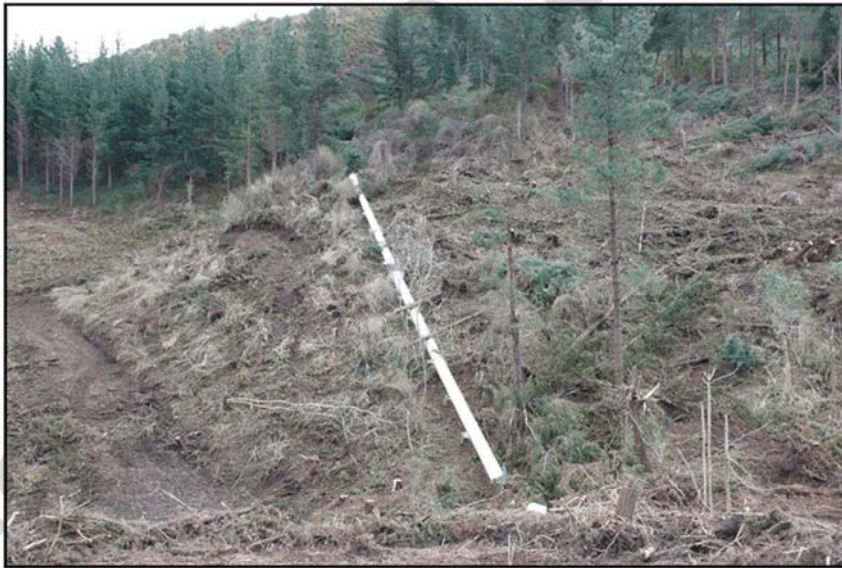
The water pipeline in Brook forest following windthrow salvage in July 2014.
